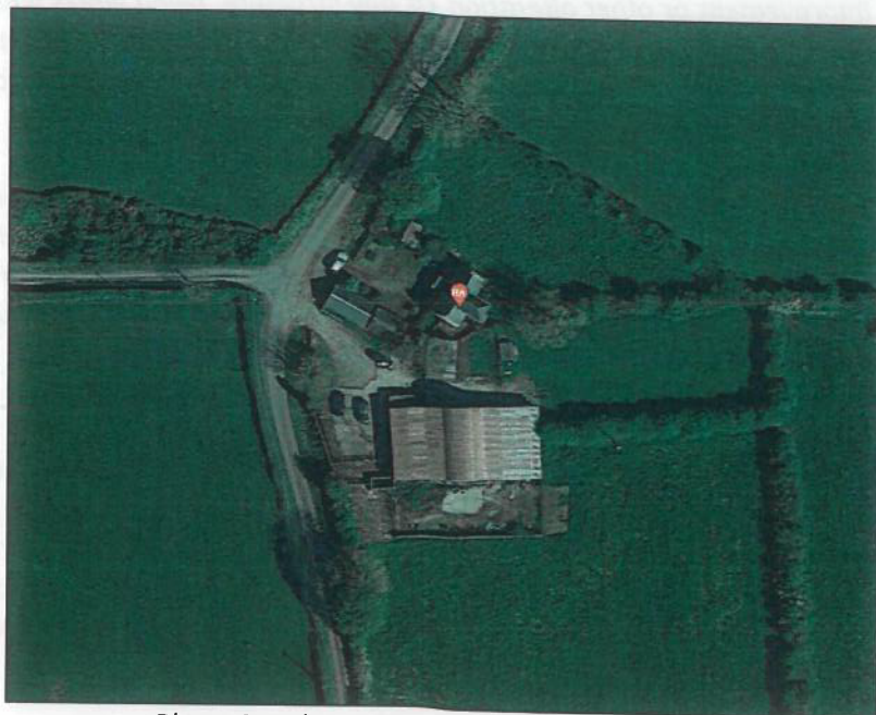
Photo 2: Subject Site (source: Google Maps).
