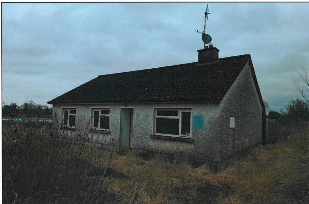
Photo 1: Front (south) elevation of existing dwelling
