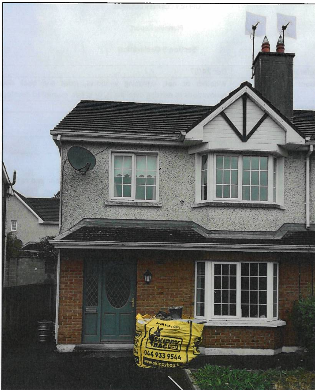
Photo 1: Front (south) elevation of existing dwelling
