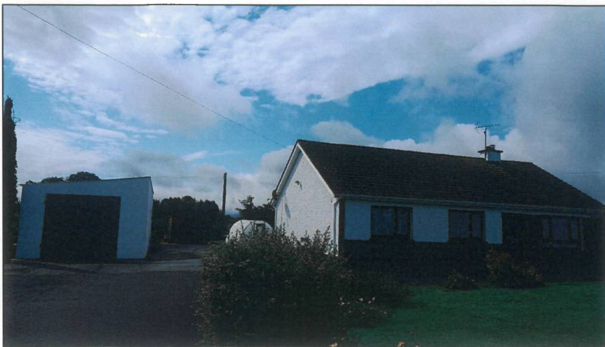
Photo 1: Front elevation of existing dwelling
