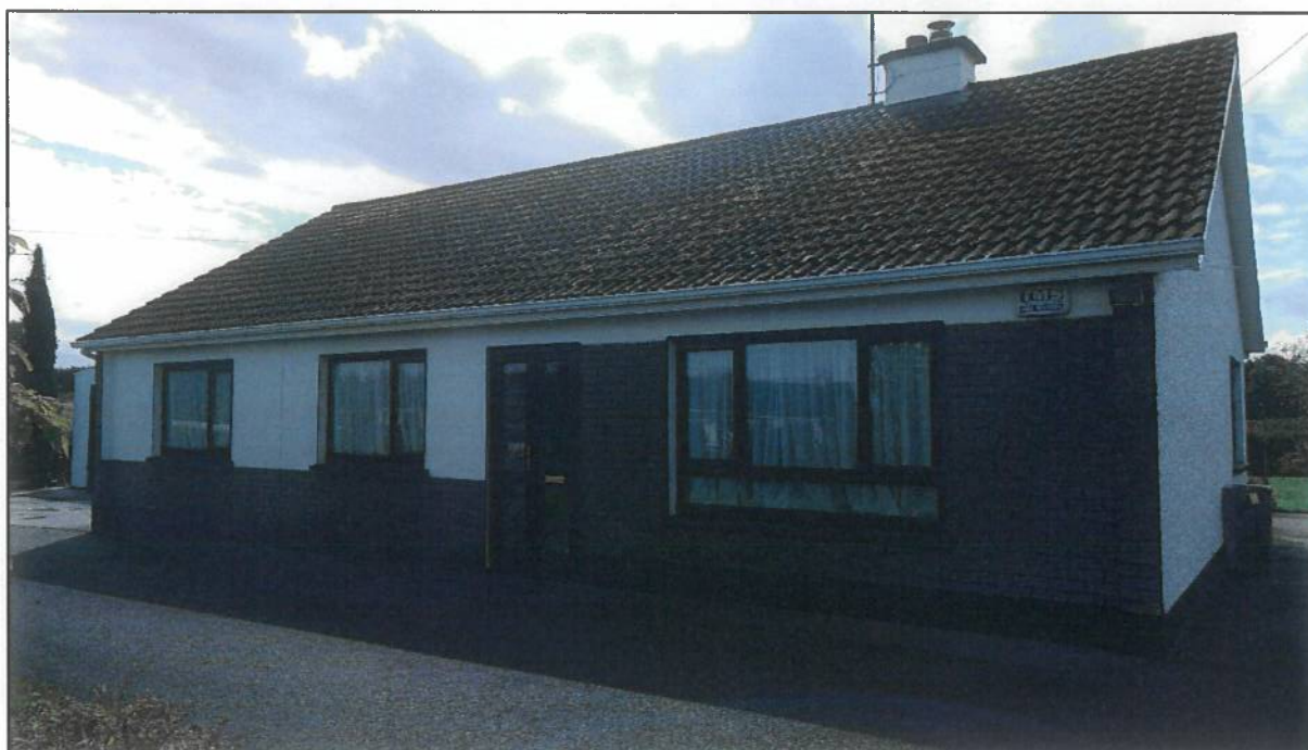
Photo 2: Front elevation of existing dwelling
