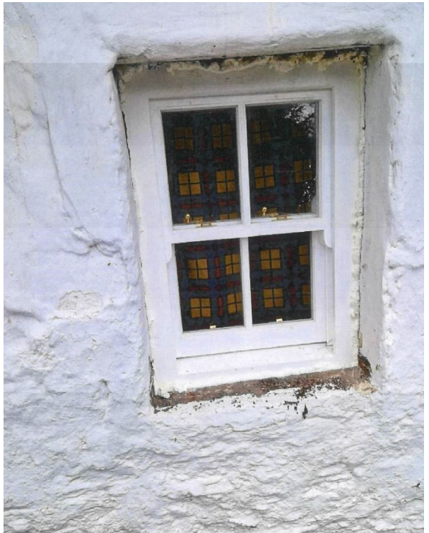
Existing casement windows removed and new timbers sash windows inserted
