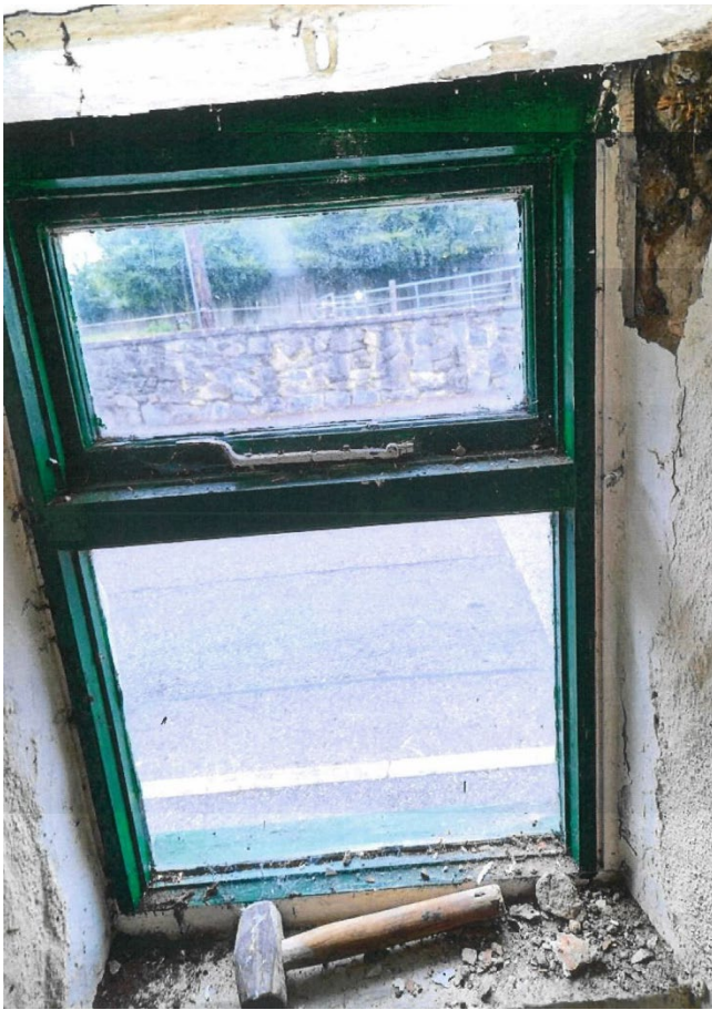
Existing casement windows removed and new timbers sash windows inserted
