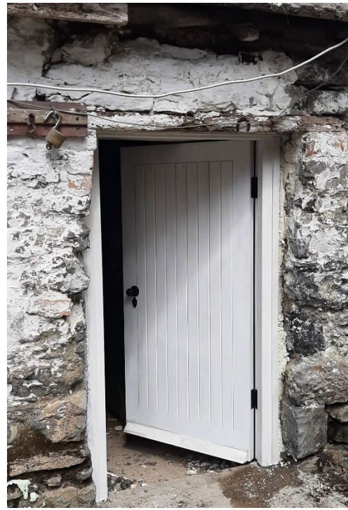
Rear door in place, lime repairs to windows surrounds (no sills)
