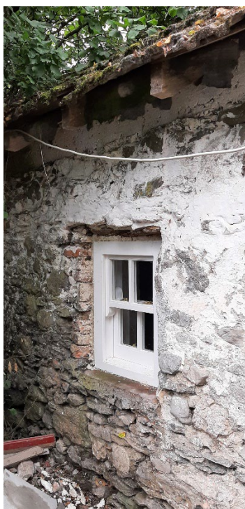
Rear door in place, lime repairs to windows surrounds (no sills)
