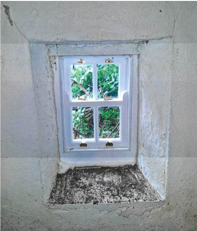
Existing casement windows removed and new timbers sash windows inserted
