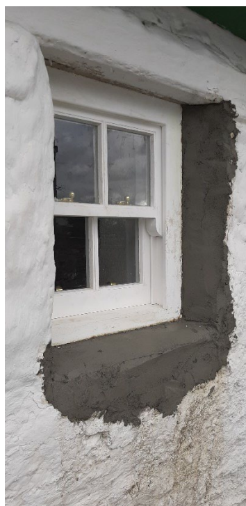
Rear door in place, lime repairs to windows surrounds (no sills)
