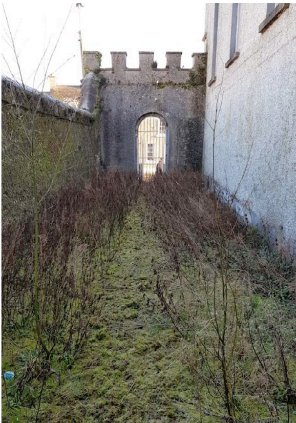
Fig 46: The judge's laneway to the north side of the courthouse
