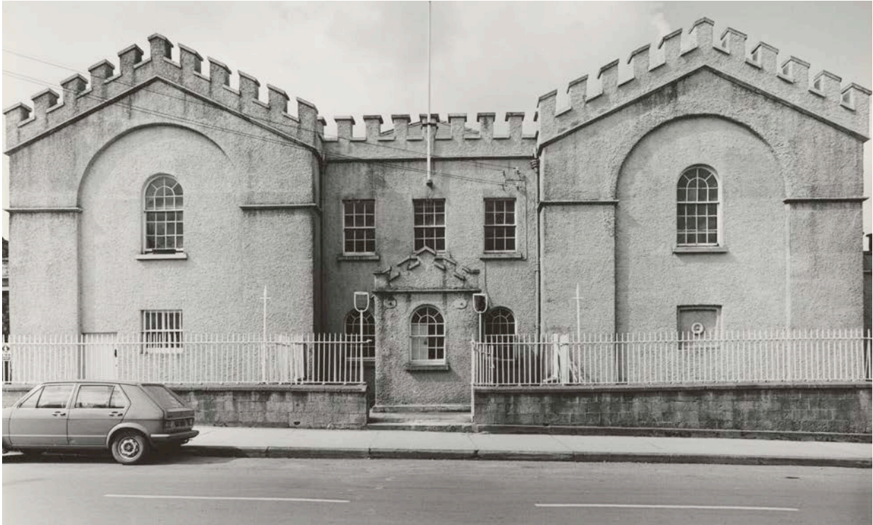
Fig 6: Birr Courthouse in 1975, with porch added to the front facade
