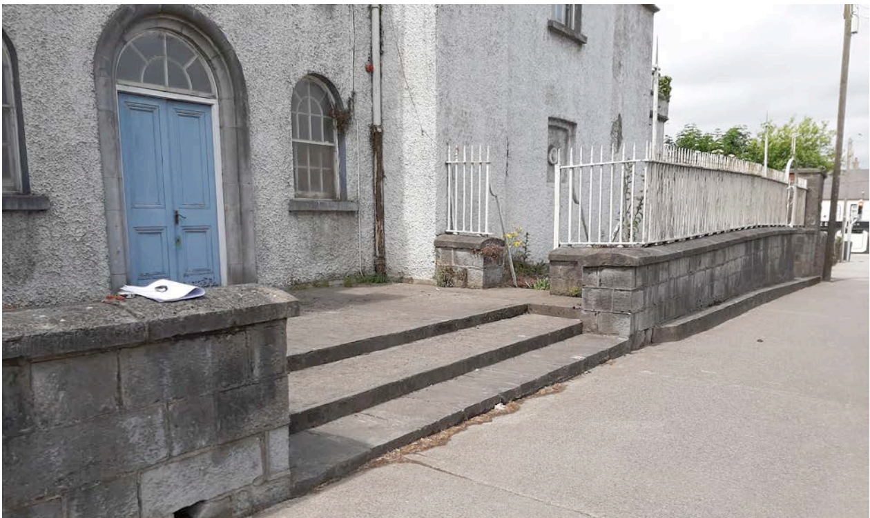
Fig 48: Front entrance steps to the Birr Courthouse
