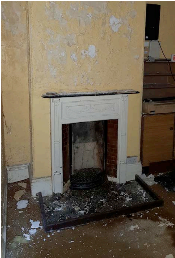
Fig 39: Cast Edwardian fireplace in the rear extension, with brick reveal
