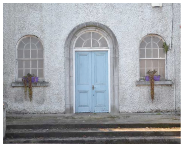
Fig 14: View of front entrance to the courthouse
