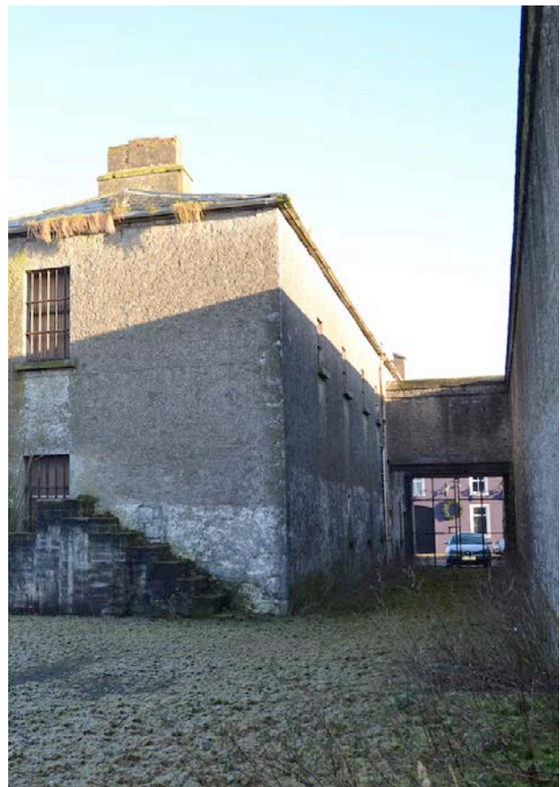
Fig 47: View down the south laneway alongside the cell block / south range
