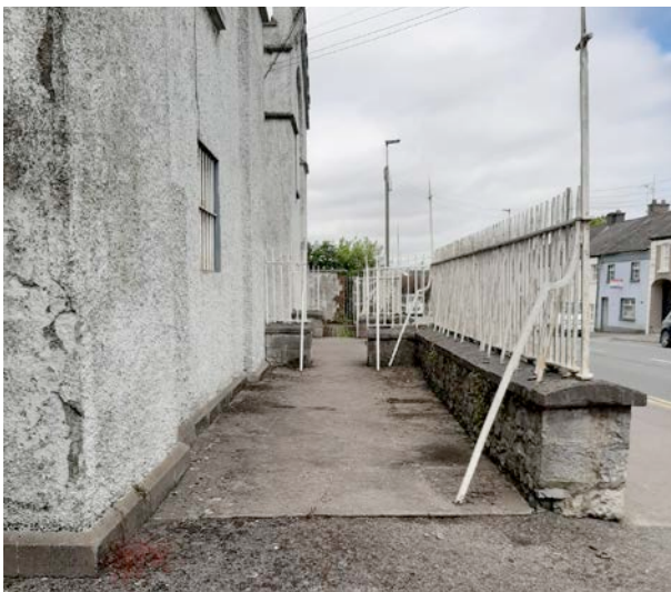
Fig 57: Ramped entry to front of courthouse
