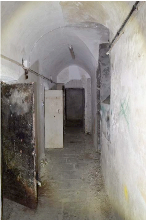
Fig 31: View of corridor down cell block with brick vaulted ceiling and stone flag floor
