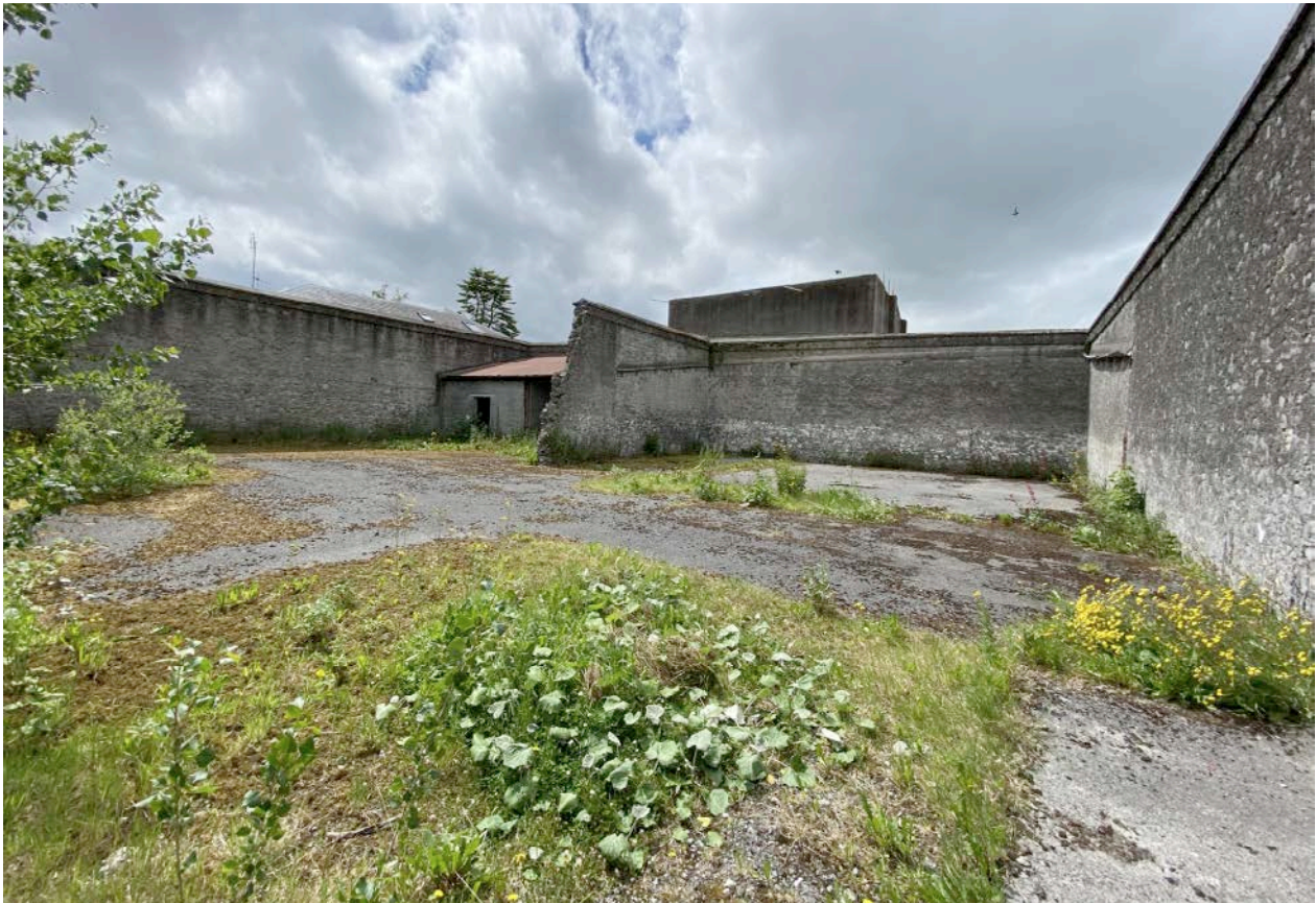
Fig 45: View of rear yard looking west, includes boundary walls
