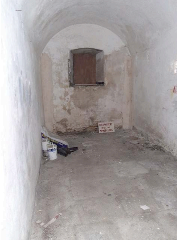
Fig 30: Plastered walls inside the cell
