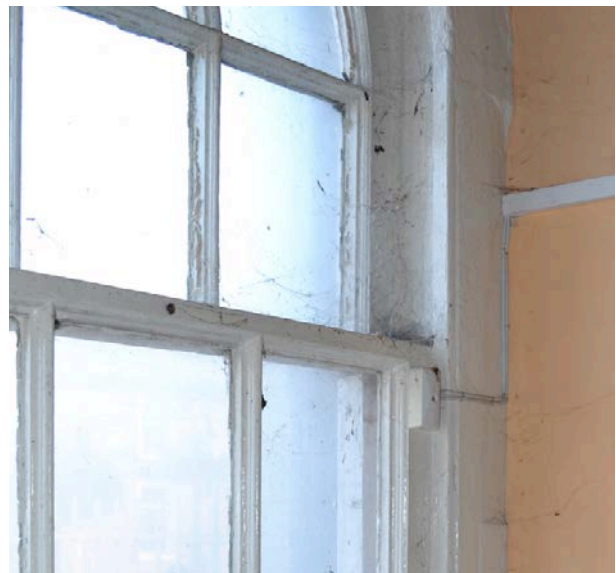
Fig 25: Historic window with lambs tongue profile on ground floor of courthouse
