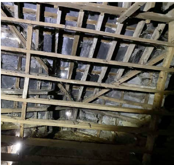
Fig 20: Underside of south range roof
