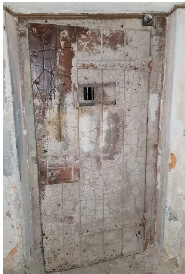
Fig 29: Original cell door with strap hinges
