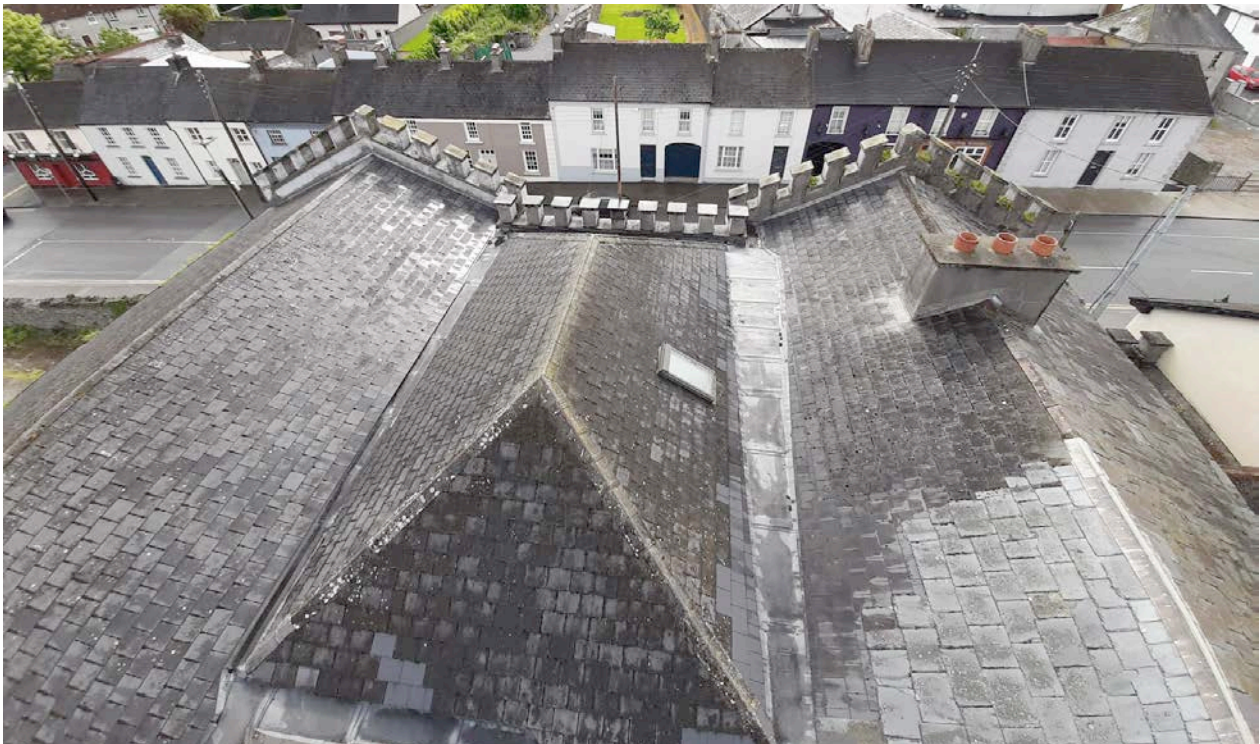
Fig 19: Photo of roofs of Birr courthouse taken from a MEWP
