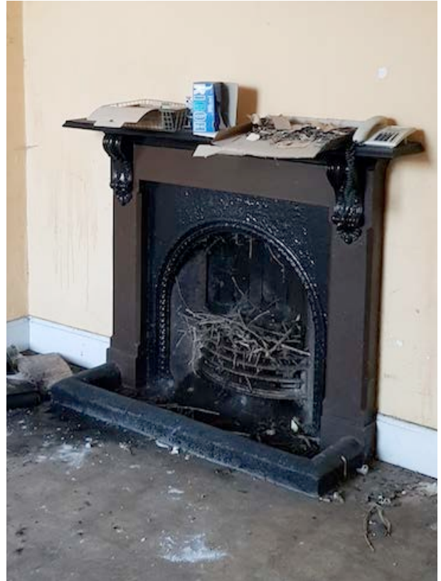
Fig 40: Painted fireplace in the front room of the south range
