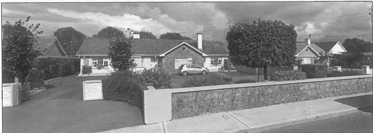
Photo 2 - Subject Site (source: Google Maps – July 2019).
