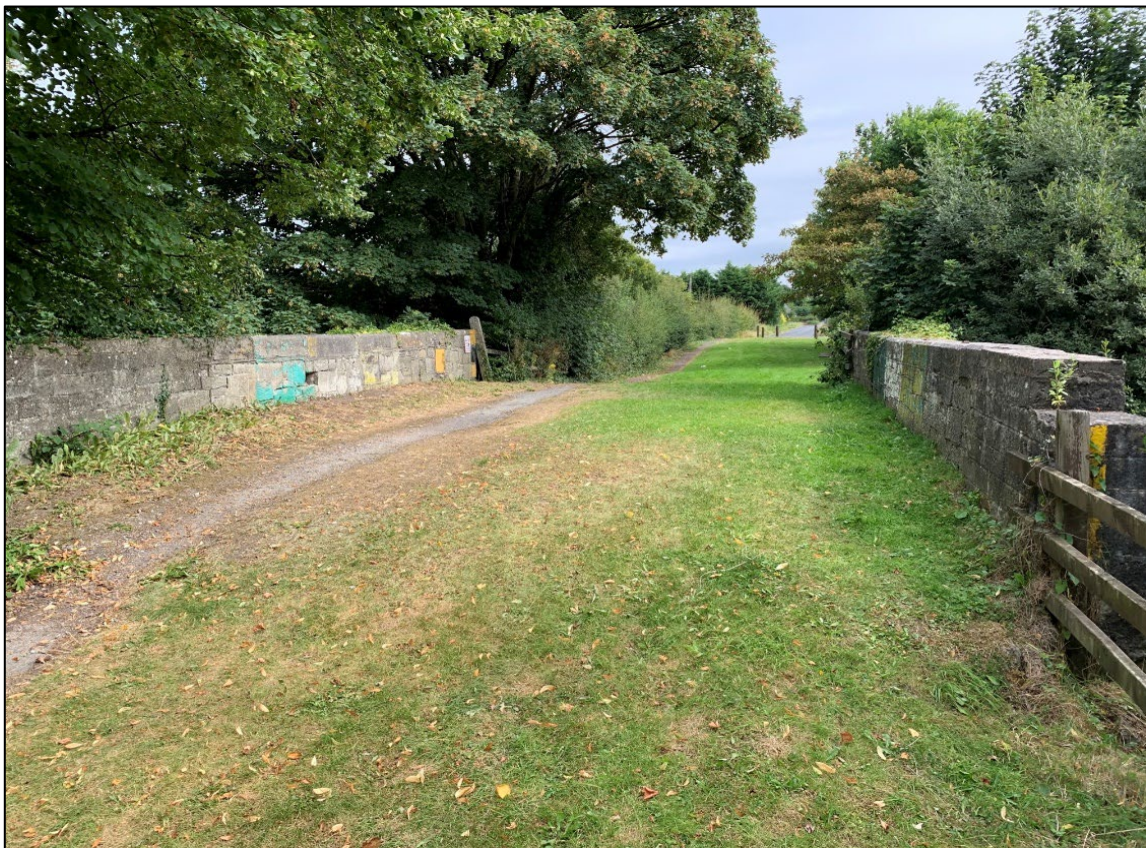
Figure 6.8 Existing pocket park at Kishowanny, Edenderry
