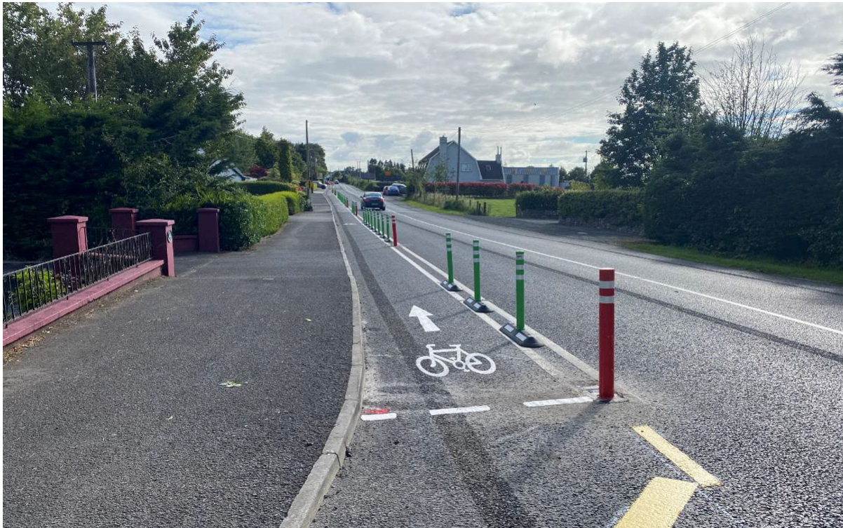
Figure 28: Segregated Cycleway on R402, July 2022
