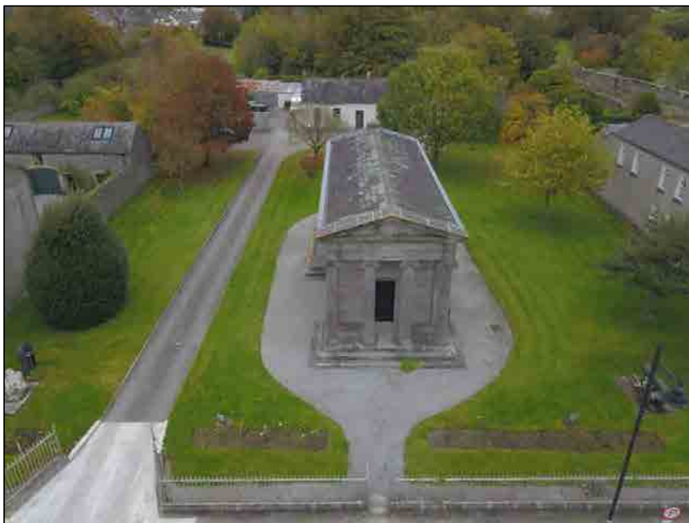
Figure 8.2 Irish Heritage School (Old Town Council Office) and St. Johns Hall
