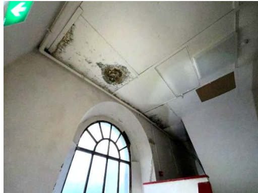
Entrance area first floor and back of Auditorium space Note staining to the ceiling behind the front elevation.
