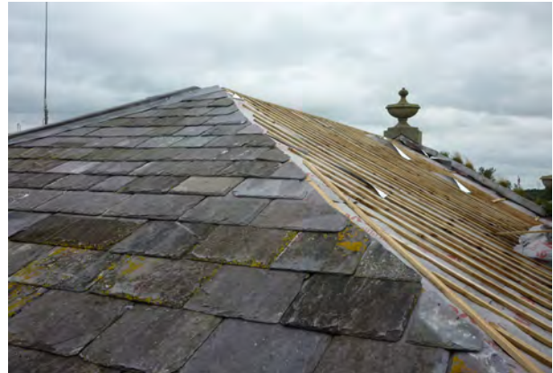
Figure 16 - View of slate roof repairs.
