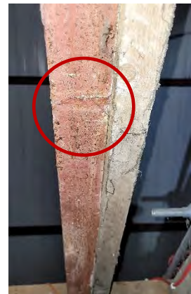
Bottom tension cord of truss has full weld across section.
