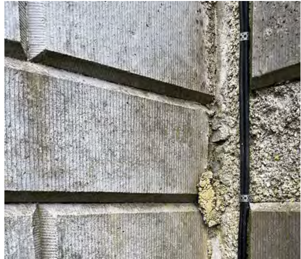
Figure 25 - View of the rusticated limestone ashlar masonry at ground floor level.
