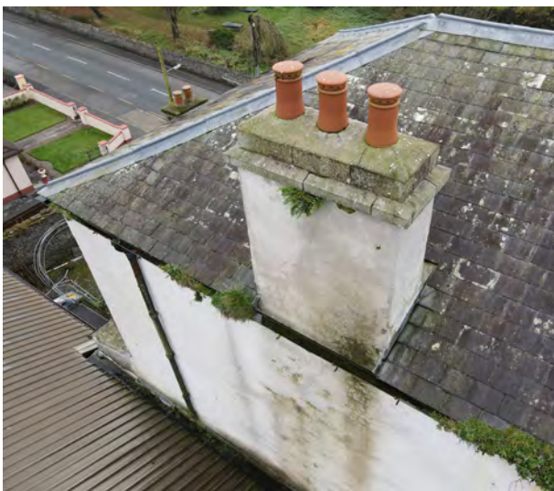
Figure 26 - View of a chimney stack with granite capping.
