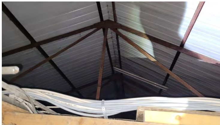
Lightweight auditorium trusses, with more recent metal sheet roofing.
