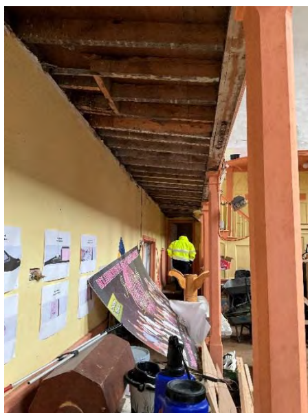
Below the courtroom in the south wing. Left detail of the underside of gallery showing extent of settlement of inboard columns
