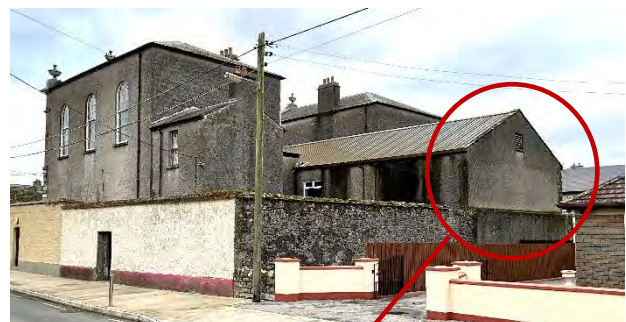
This wall replacement may require the dismantling of boundary wall down to ground level.
