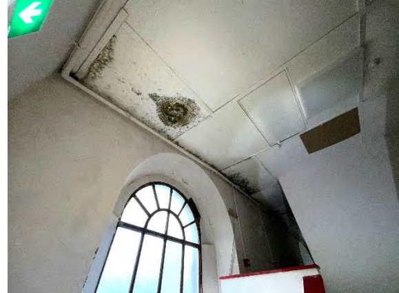
Front central window Notice staining to ceiling.
