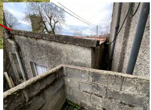
View onto end elevation and roof of former fire station. Note gap to historic structure and insubstantial 100mm block parapet to escape stair.
