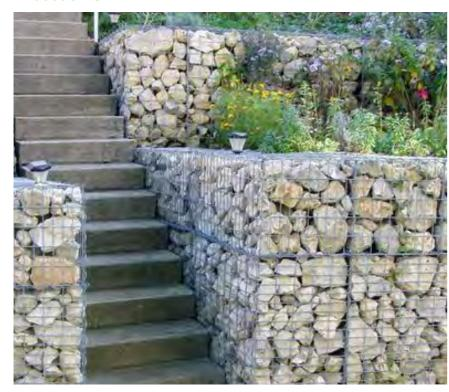
Tiered seating using gabions filled with reclaimed demolished site material and faced with local stone. Planting will create a soft frontage to the newly renovated and extended Convent.
