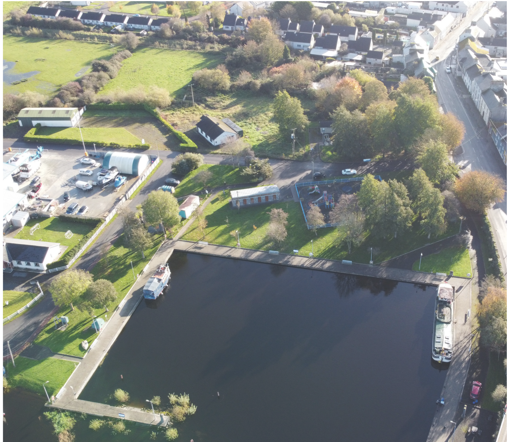
Figure 2.10 Banagher Marina and Environs - Aerial View
