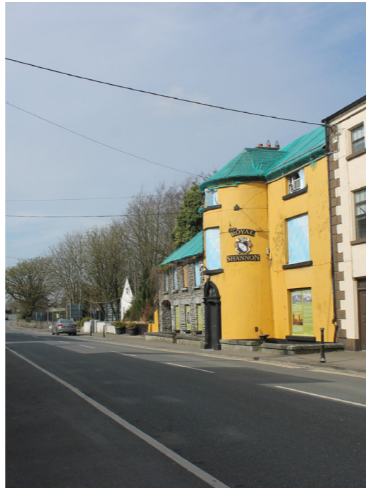
Figure 2.9.1 Banagher Marina and Surrounding Context
