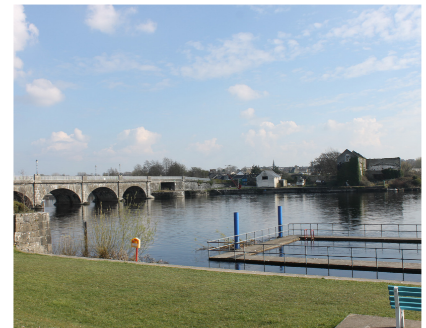
Figure 2.9.4 Banagher Marina and Surrounding Context
