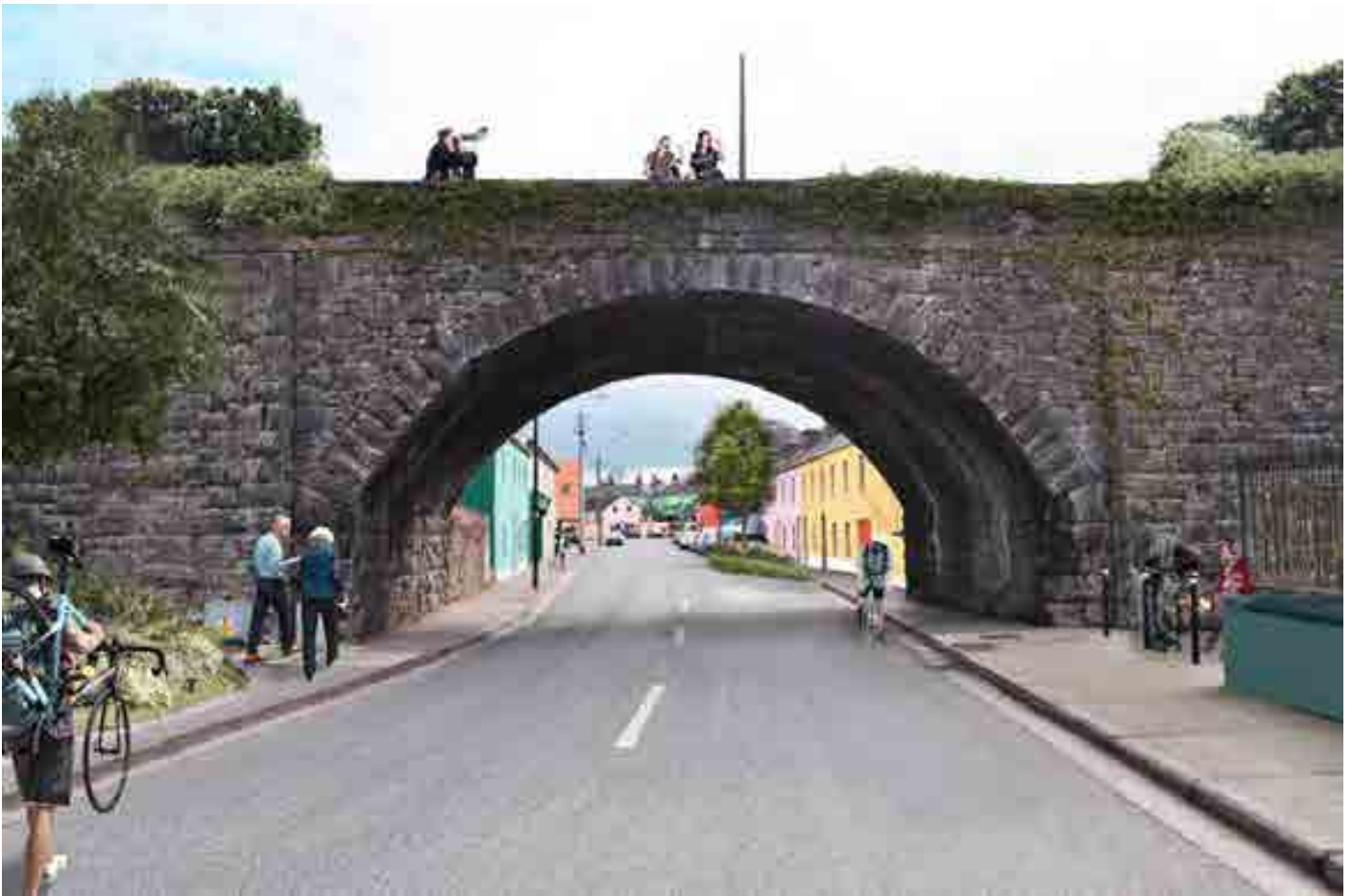
Figure 4.18 Future Railway Greenway link on River Street
