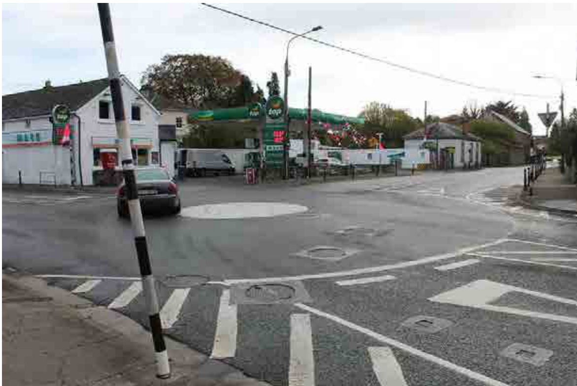
River Street / Kilbeggan Road Roundabout - substandard pedestrian facilities (no crossings and narrow footpaths)
