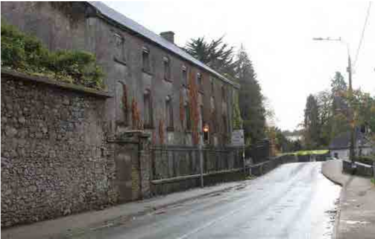
Charlestown Bridge (lack of footpath on eastern side)
