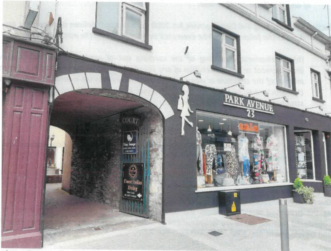
Plate 1: Image of existing shop front
