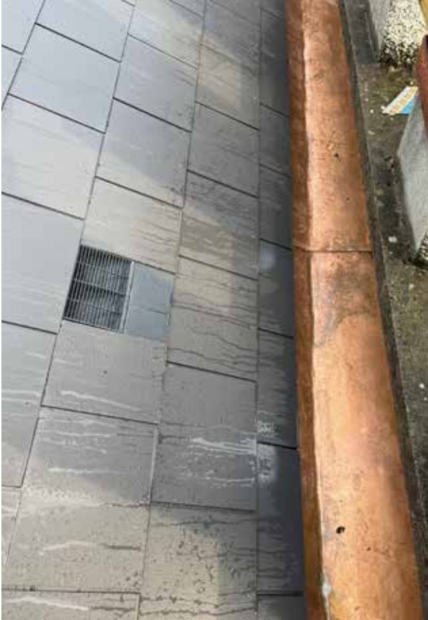
Copper Parapet Gutter - Upon completion of works.
