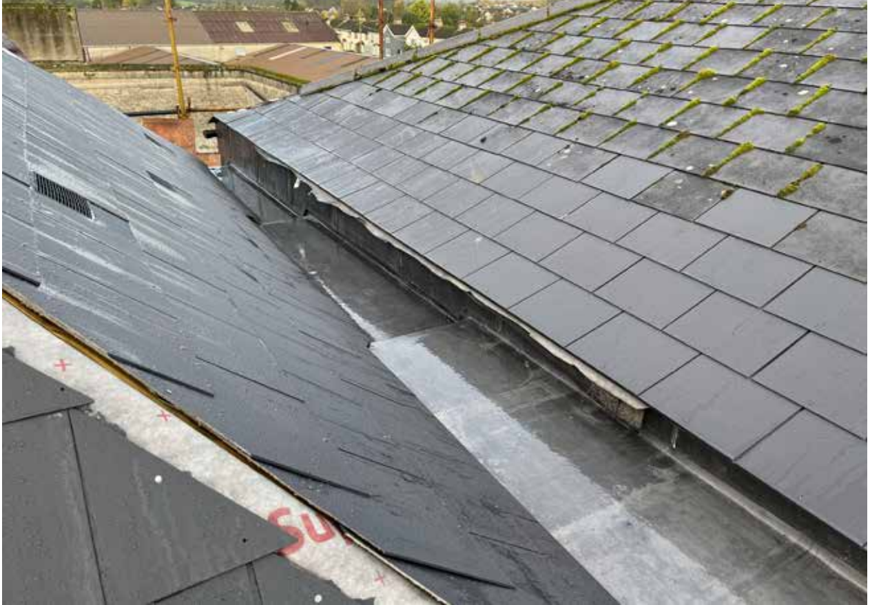
Lead Valley / Gutters 3&4 - Upon completion of the works.
