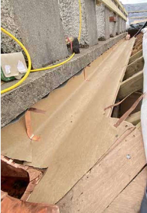
Copper Parapet Gutter - Before & during works being carried out.
