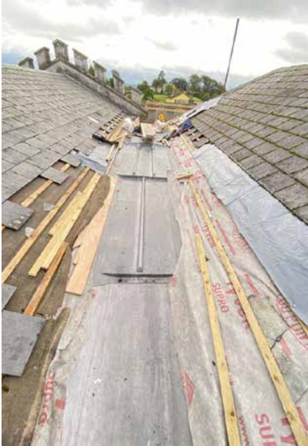
Lead Valley / Gutter 2 - Before & during the works.
