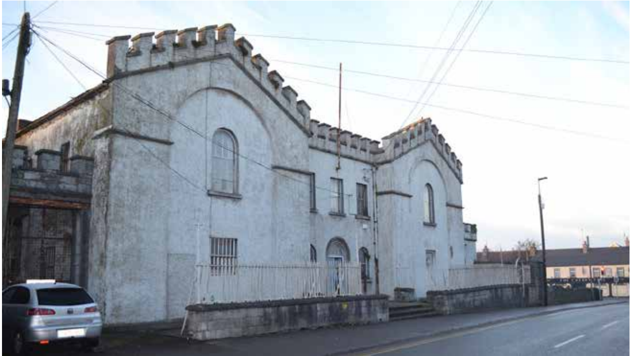
Birr courthouse prior to commencement of works on site
