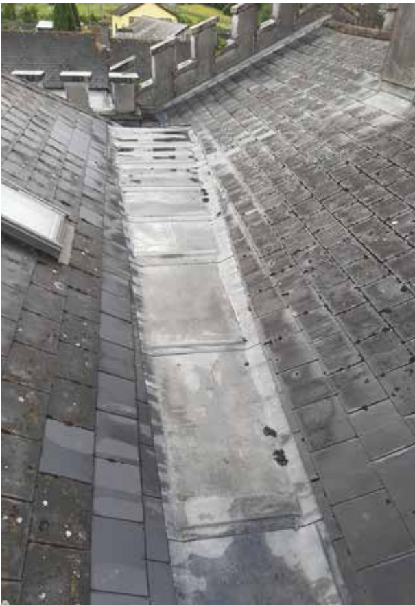
Lead Valley / Gutter 1 - Before works were carried out.
