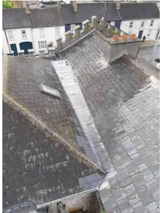
View of the leadwork valley between the south range and central range
