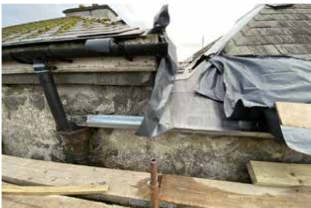
Lead Valley / Gutters 3&4 - Before works were carried out.
