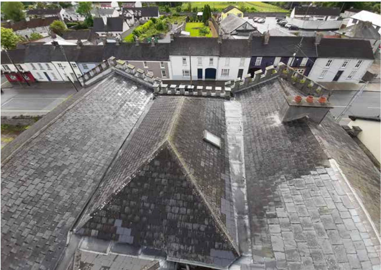
View of the roofs from the MEWP
