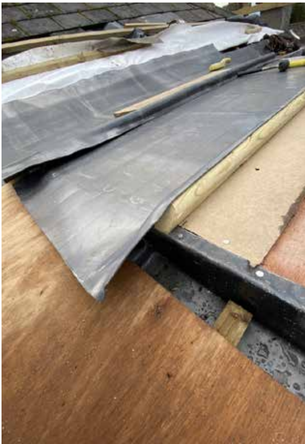
Lead Valley / Gutter 1 - During works being carried out.
