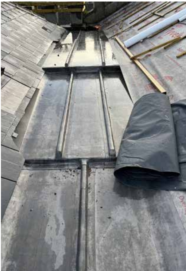
Lead Valley / Gutter 1 - Upon completion of works.
