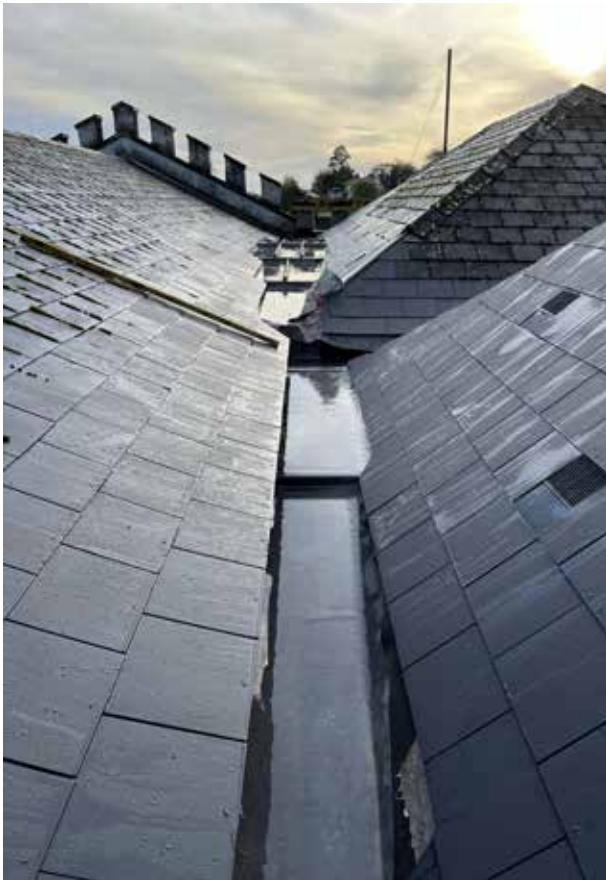
Lead Valley / Gutter 2 - Upon completion of works.
