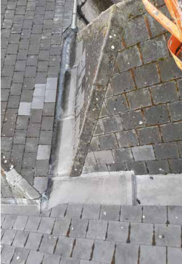
Lead Valley / Gutters 3&4 - Before works were carried out.
