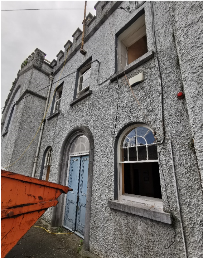
2021_0917 – Windows repaired and refitted by Core Joinery
