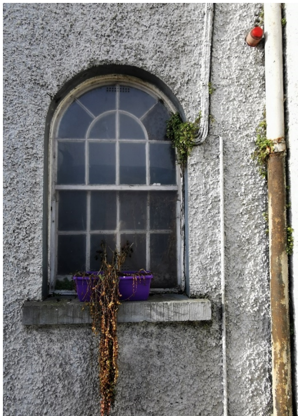
Survey of existing front facade windows
