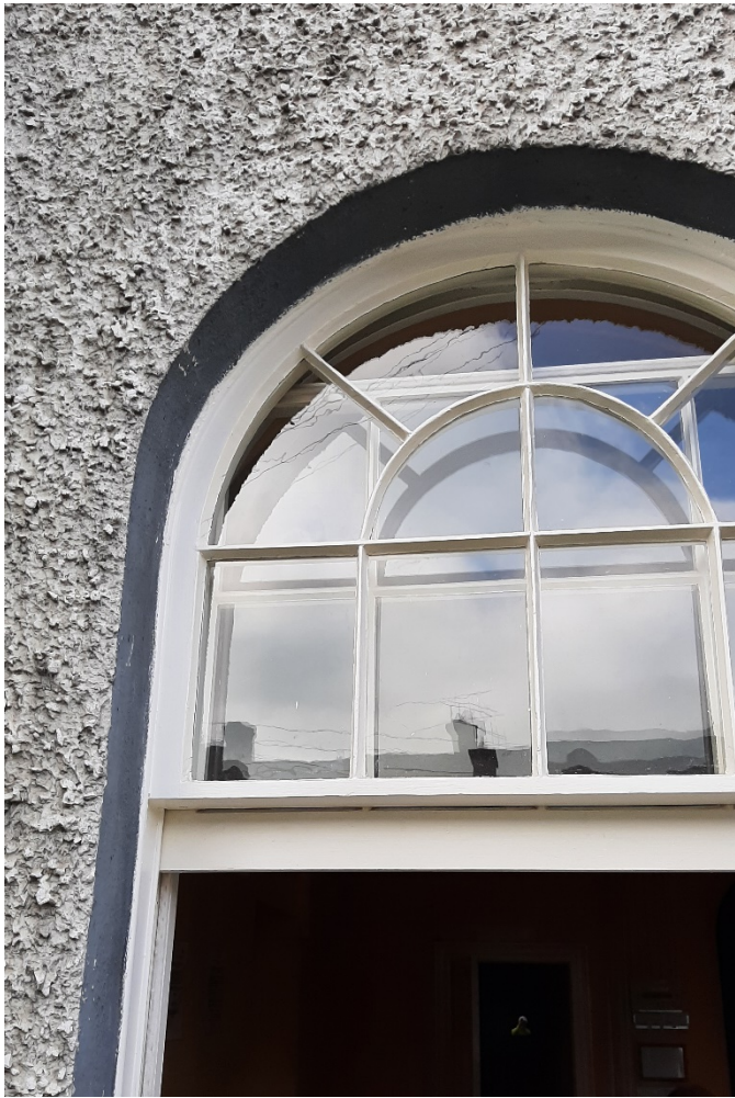
Entrance lobby with upper historic sash repaired, replacment lower section with matching glazing detail
