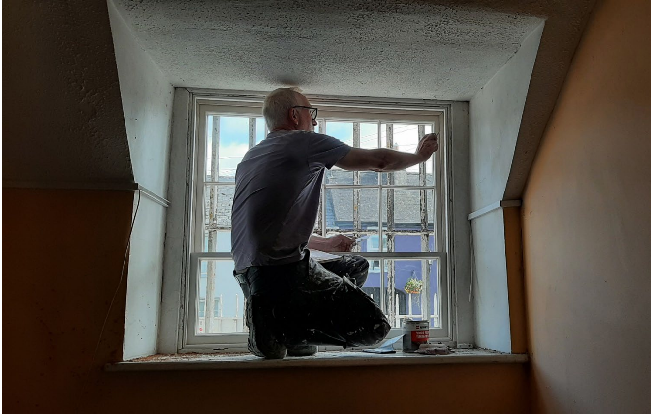
8/4 sash window and large courtroom sash – final coat of paint
