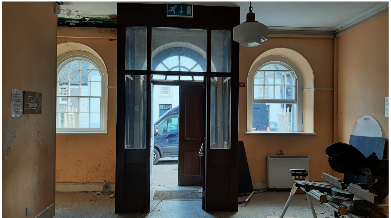
Entrance lobby with upper historic sash repaired, replacment lower section with matching glazing detail
