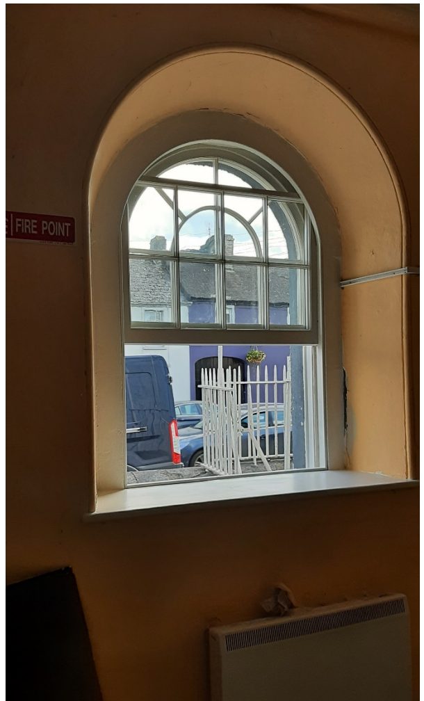
Entrance lobby with upper historic sash repaired, replacment lower section with matching glazing detail
