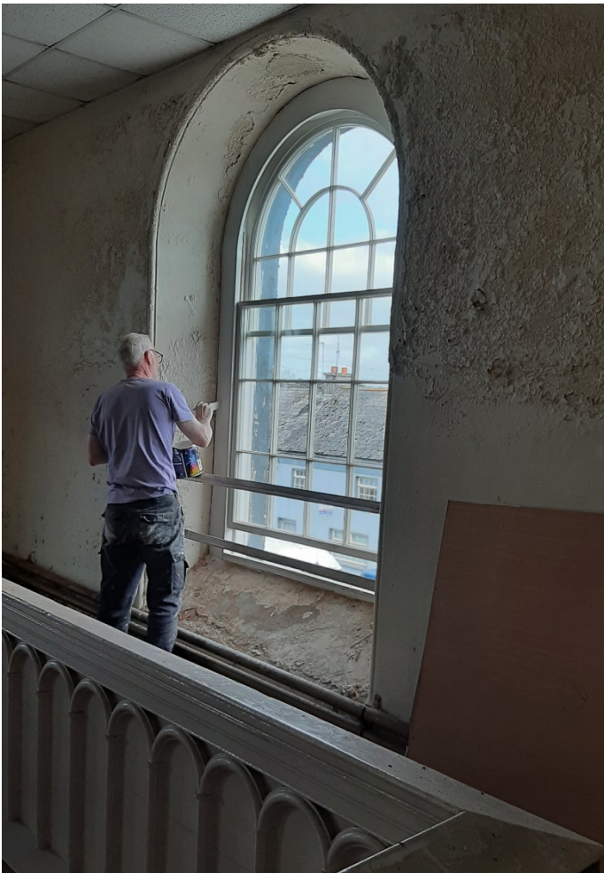
8/4 sash window and large courtroom sash – final coat of paint
