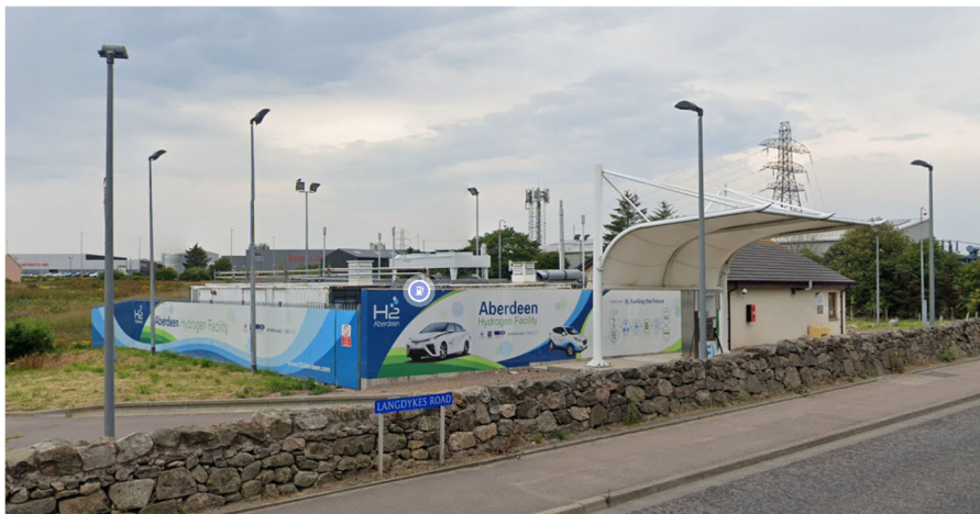
Figure 4-19: Aberdeen City Hydrogen Energy Storage (ACHES)
